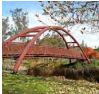
An Adirondack-style bridge would greatly enhance the main gateway into Brant Lake Hamlet.
